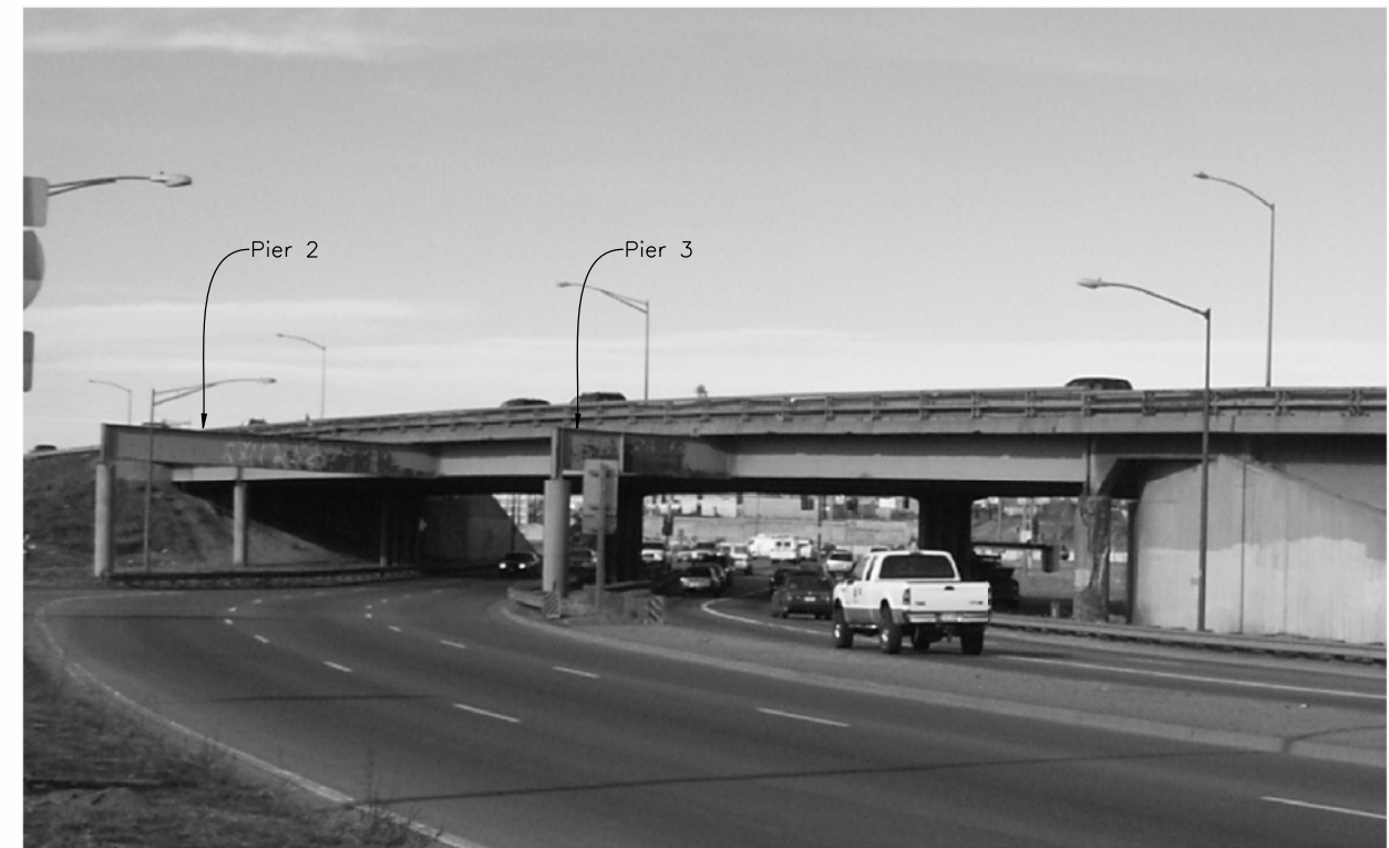
EXISTING STRUCTURE F-16-DT (Looking North)
